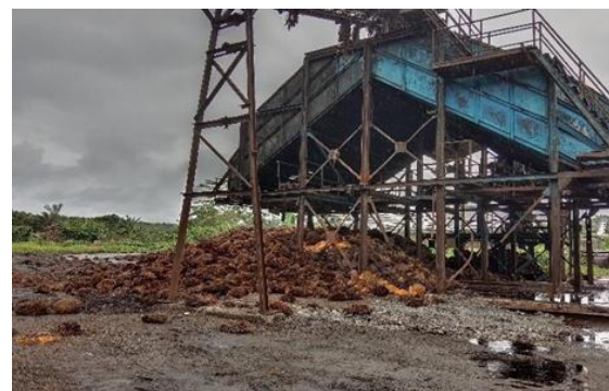
Figure 10. Empty Bunch Hopper Station (Source: Personal Documentation)
